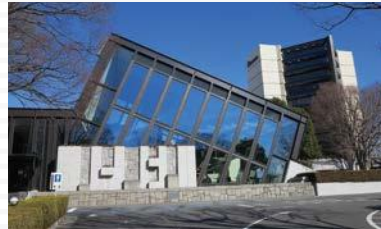
Renovation of lounge building—addition of temporary evacuation site in the case of disasters
